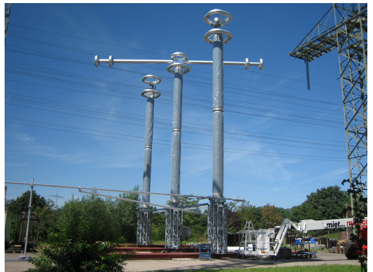
Fig. 3: 800 kV disconnector
