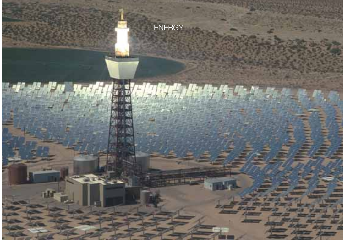
Figure 7 Solar II central receiver plant in Barstow, California (Source: SNL)
