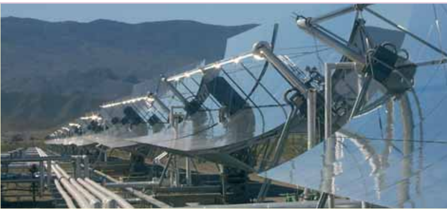
Direct steam generating parabolic trough of the DISS project at Plataforma Solar de Almeria, Spain
