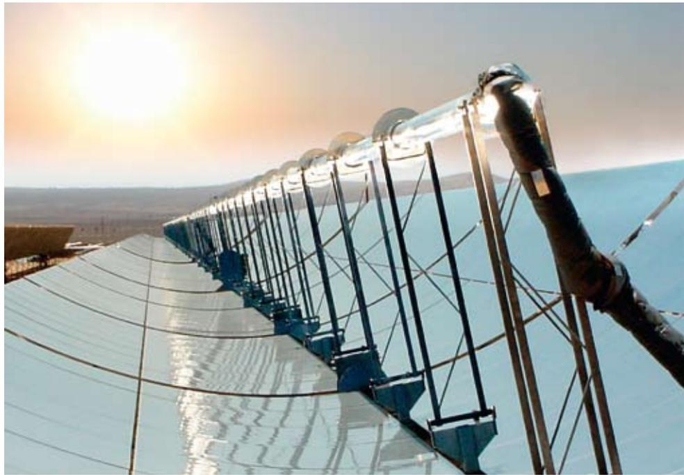
*Close up view of parabolic trough and heat collector.*
