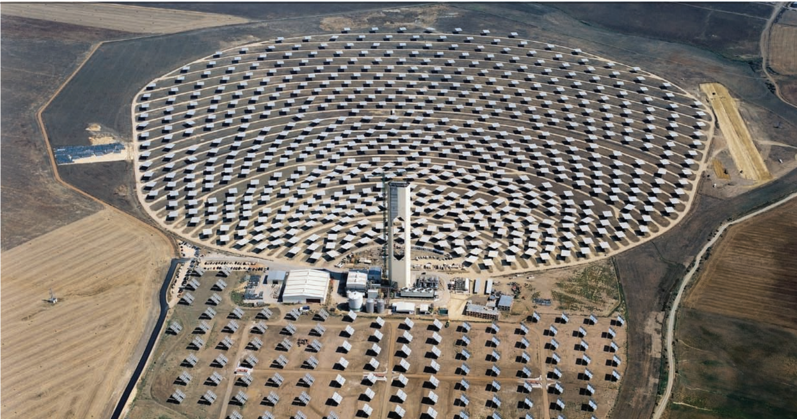
Europe's first commercial concentrating PS10 solar power tower is operating near the sunny southern Spanish city of Seville. The 11 MW solar power tower produces electricity with 624 large movable mirrors called heliostats.
